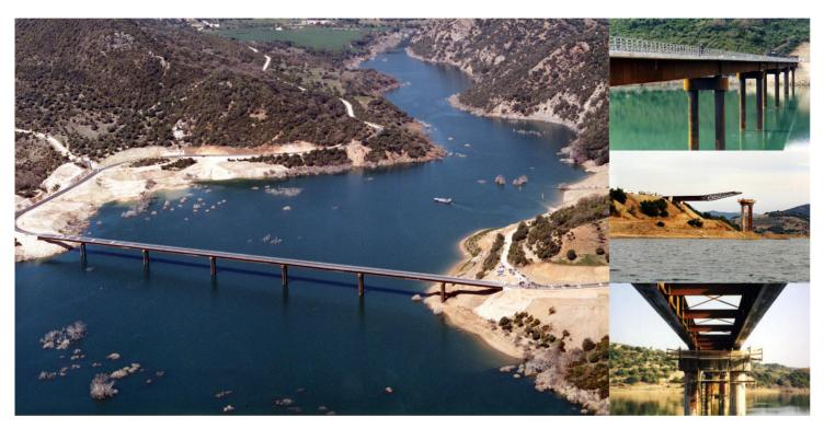
The Picado Bridge has a total length of 450.0m and a total depth of 2.30 m. Its longest span has a length of 70.0m. The deck is composed of two steel girders. The upper concrete slab has been cast over pre-cast slabs placed over the girders. The piers consist of two 1.60m diameter pile-columns which vary in height between 23.0m and 35.0m. The head of the piers is composite with the steel box section being used as framework and reinforcement.
